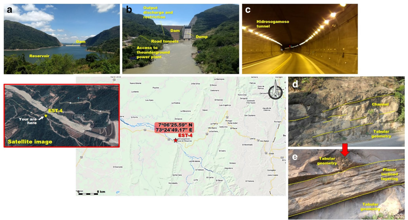
Fig. 6 (a)–(b) Panoramic view of the Sogamoso Hydroelectric Power Plant. (c) Hidrosogamoso tunnel along the Bucaramanga-Barrancabermeja highway. (d)–(e) Outcrops of conglomerate sandstones of the La Paz Formation on the left side of the highway.
